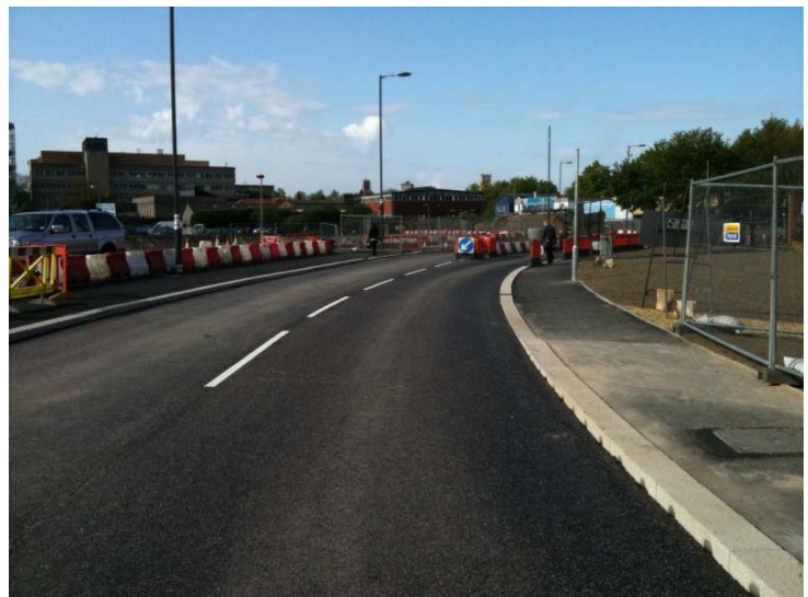
New link road looking south west towards Pitt Street
